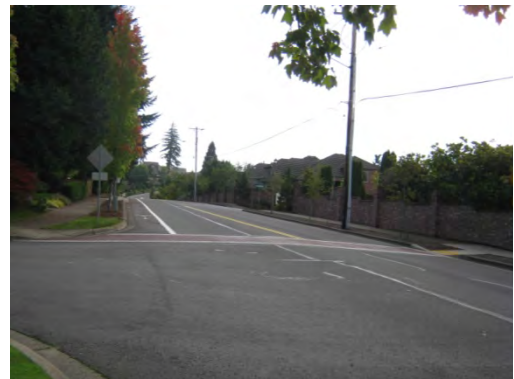
Unsignalized crosswalk on SW 108th Avenue
