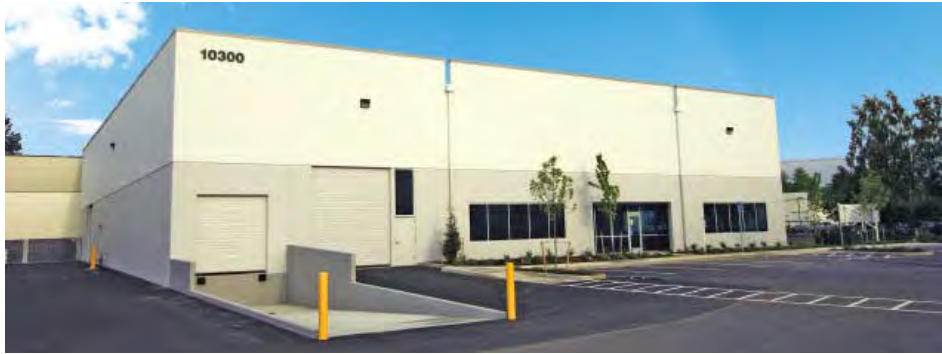
Figure 29 Example of typical flex industrial building, located in Tualatin.
