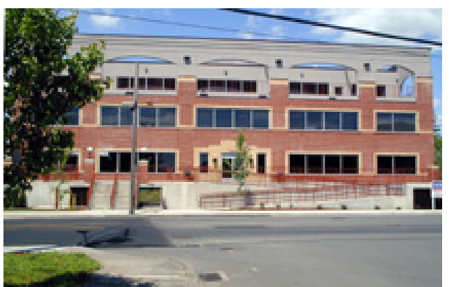
Aspen Place – Boones Ferry Road
