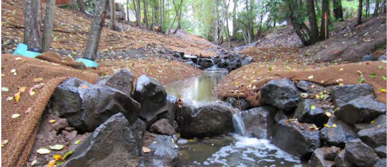
Photo 2. Otak photo of newly constructed Saum Creek channel in Chieftan/Dakota Greenway (c. 2013)
