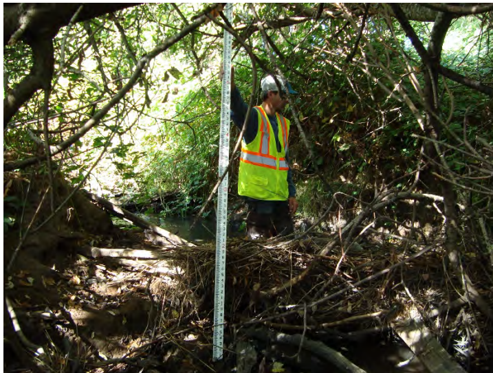
Site location: South of Sequoia Drive Photo number: S2-12 Description: Debris jam
