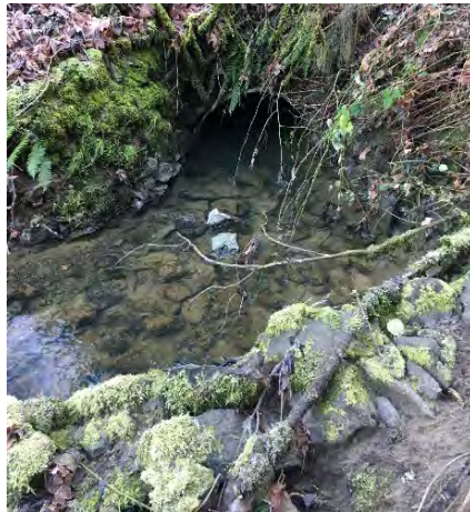
Image 1. Downstream end of culvert with rock/concrete wall for erosion prevention
