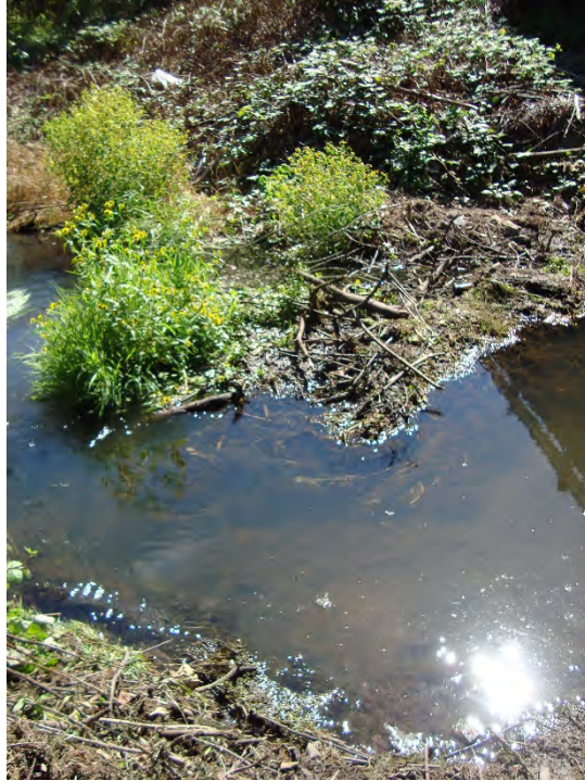
Site location: Nyberg Creek on downstream side of SW 65 th Ave. Photo number: N1-11 Description: Photo taken from left bank (north side) on 9/12. Additional debris was removed between 9/11 and 9/12. See photo N1-12 for comparison.
