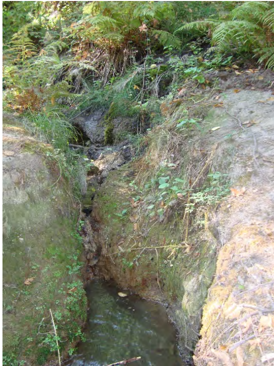
Site location: 750' upstream of SW 105 th Ave. Photo number: H3-10 Description: Side channel, left bank, deep incision, looking downstream
