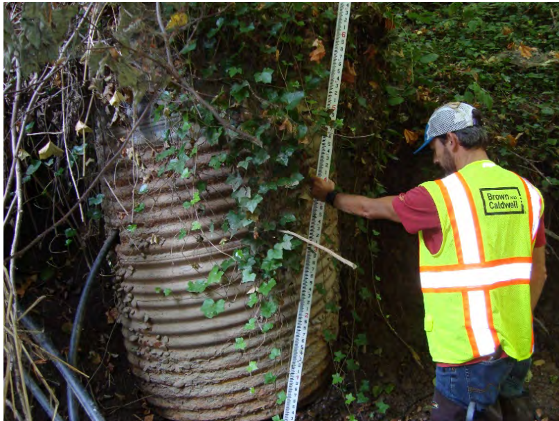
Site location: ~400' upstream from Tualatin River Photo number: S1-4 Description: Corrugated steel pipe (former water intake?) on left bank
