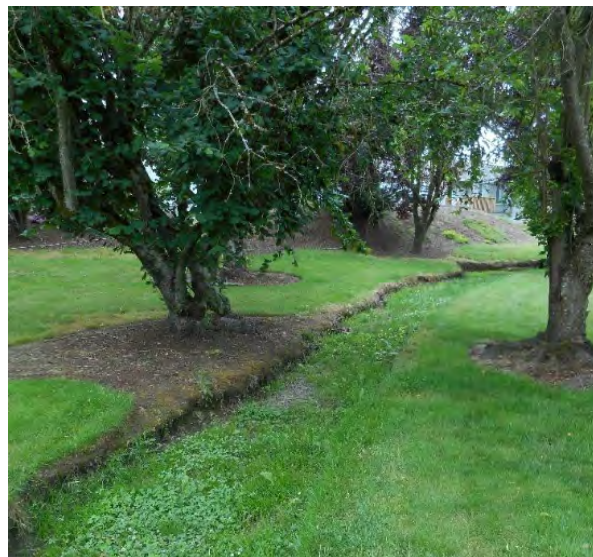
Image 1. Incision and sloughing in the open channel
