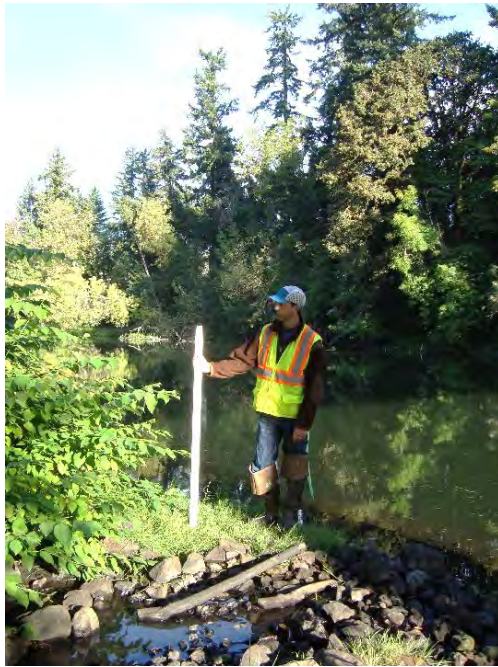
Site location: Mouth of Hedges Creek below Boones Ferry Road bridge at Tualatin River Photo number: H1-1 Description: 3" to 1.5' rocks in channel (rip-rap stabilization)
