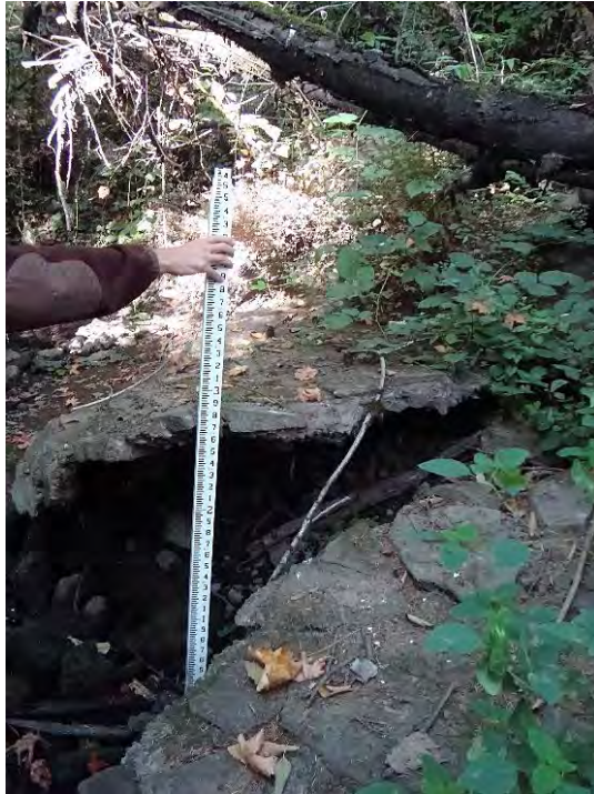
Site location: 200' upstream of Tualatin River Photo number: H1-5 Description: Concrete poured in channel from left bank
