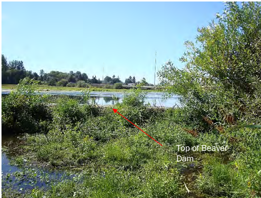
Site location: Downstream side of beaver dam Photo number: N2-5 Description: Dam extends the entire length of valley bottom, creating a ~3 - 4' drop
