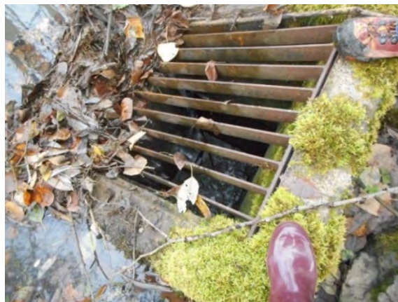
Image 2. Existing pond outfall control structure
