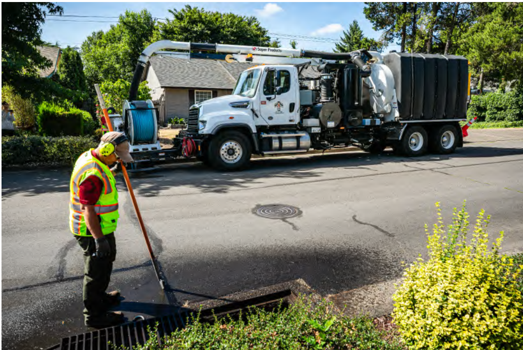
Storm System Cleaning
