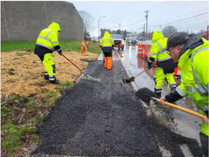
Temporary Asphalt Sidewalk Installation
