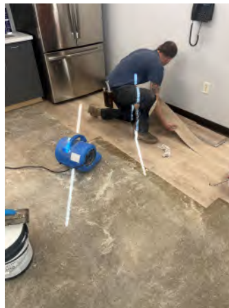
Police flooring replacement
