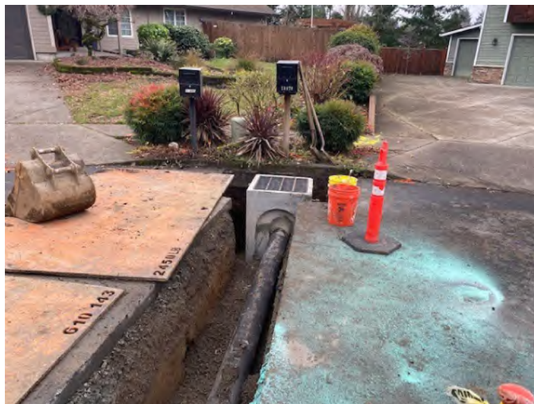
Stormwater repair
