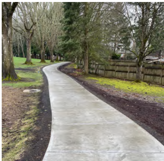
Boones Ferry Road Sidewalk Improvements
