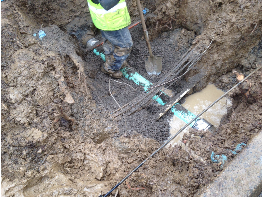
Sewer Lateral Repair
