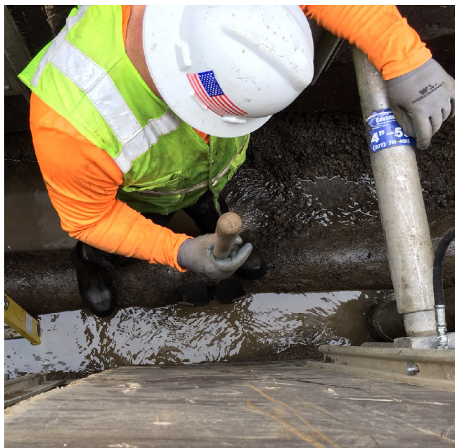
Sanitary Sewer Main Line Repair
