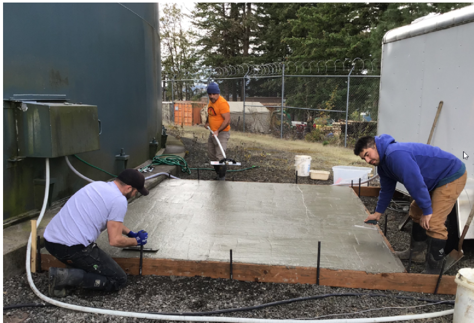
Pouring concrete at water reservoir
