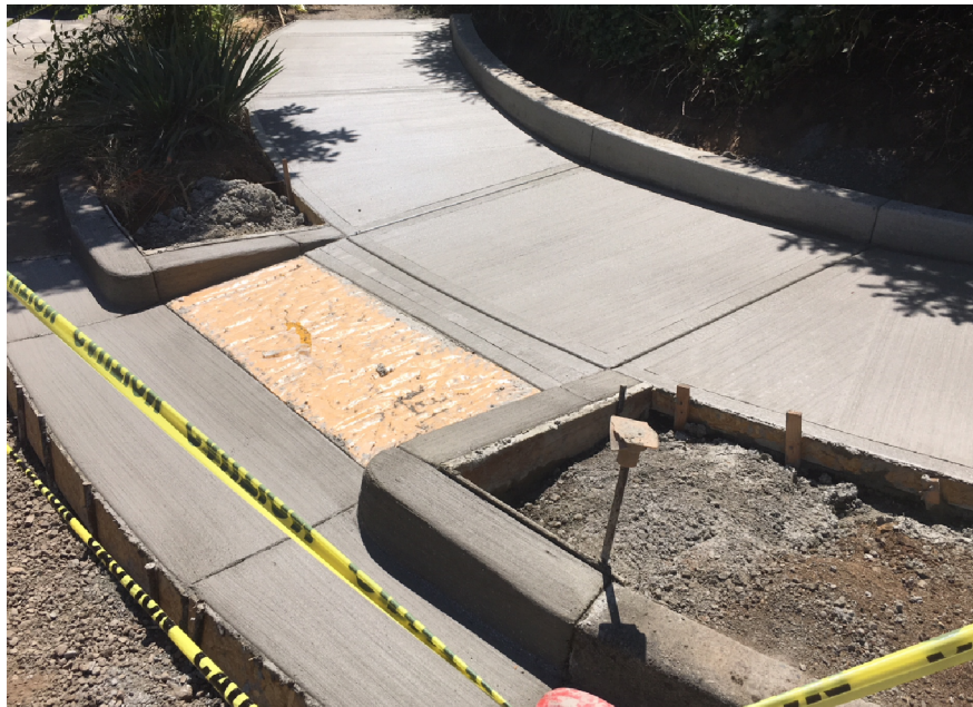
Road Utility Work
