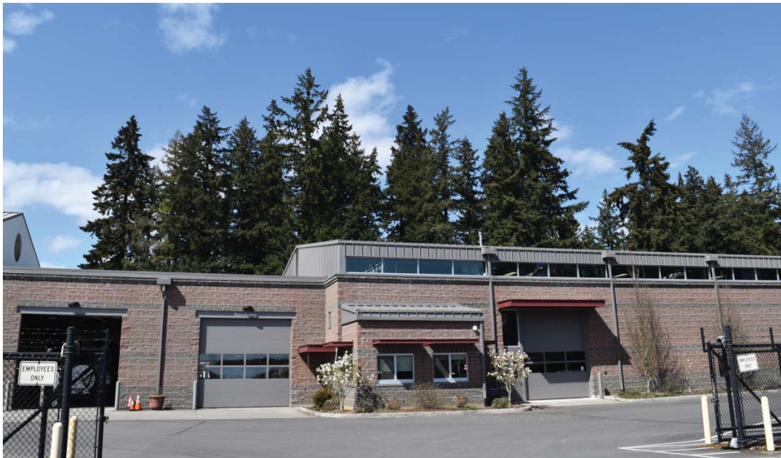
City Fleet and Warehouse Facility
