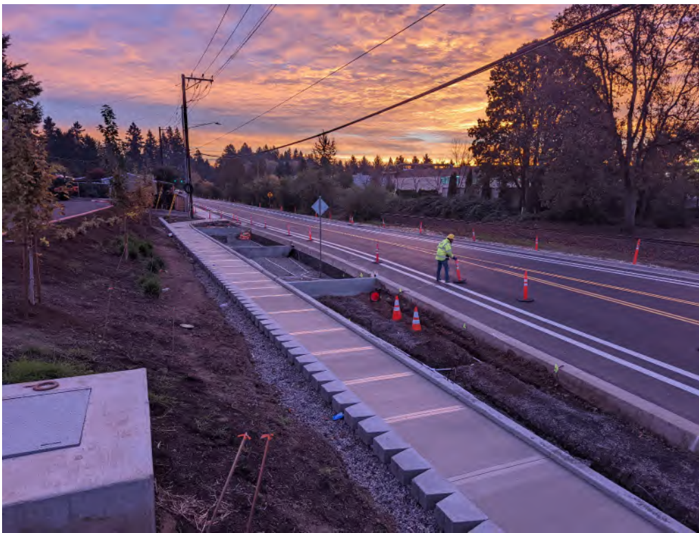
Herman Road Project
