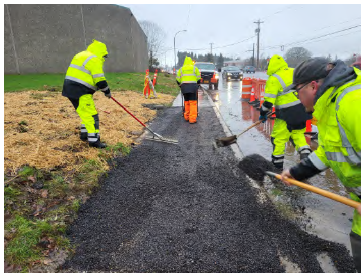
Temporary Asphalt Sidewalk Installation
