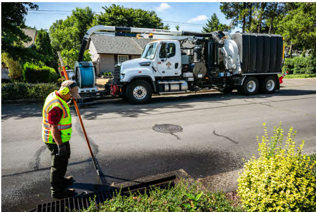
Storm System Cleaning
