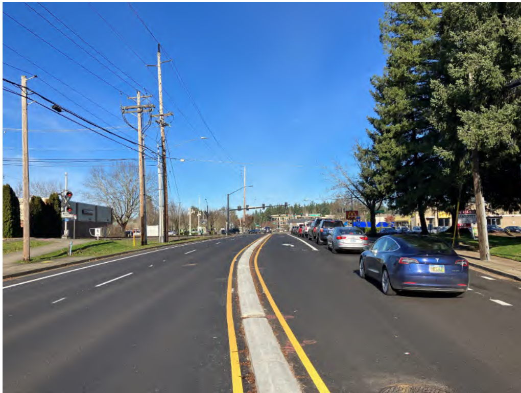
Boones Ferry Road Improvement
