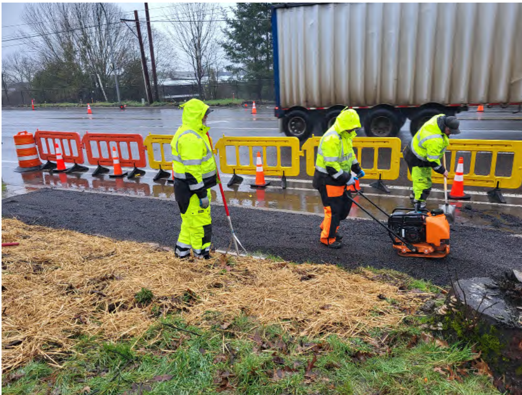
Installing Temporary Asphalt Path after Sewer Lateral Repair
