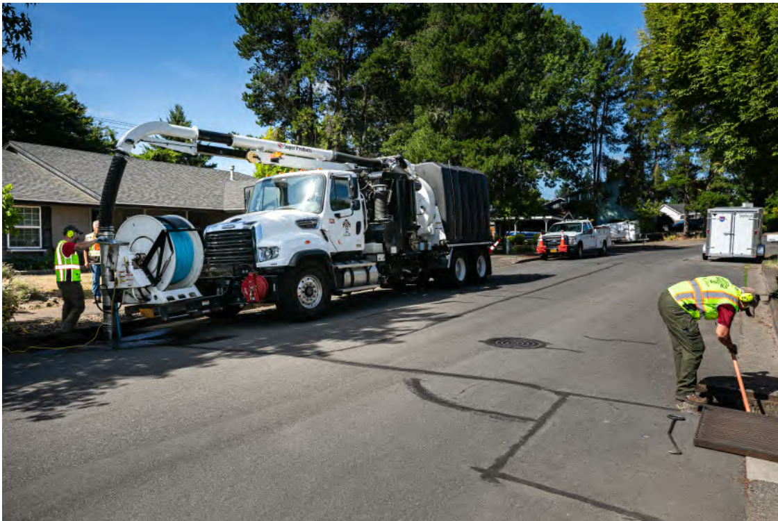
Storm System Repair
