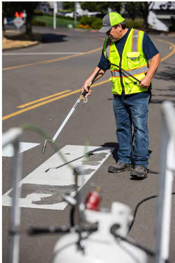
Road Markings Repair
