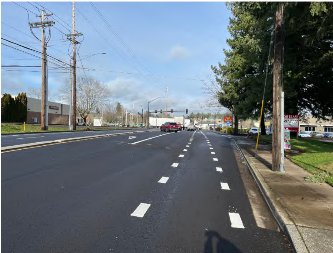
Boones Ferry Road Transportation Project
