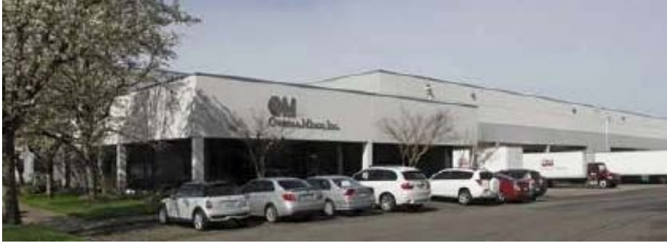
Figure 28 Example of typical building with a mix of office space and warehouse/distribution space.
