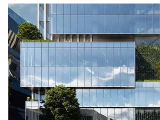
4 STOREFRONT / CURTAIN WALL GLAZING SYSTEM
