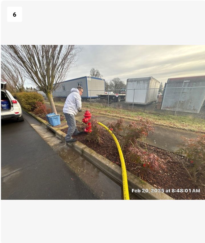
Ernie Castro of City of Tualatin operating the hydrant valves.
